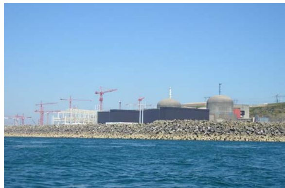
Flamanville Nuclear Power Station
