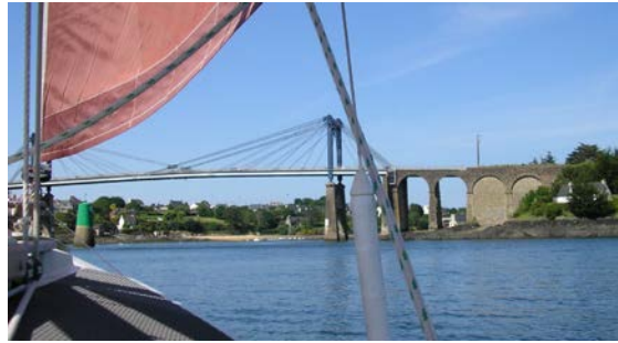
The bridge at Lézardrieux
